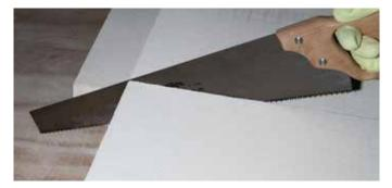
The KÖSTER Hydrosilicate Boards are cut using a common saw. Alternatively, the boards can be cut with a utility knife drawn along a steel edge.
