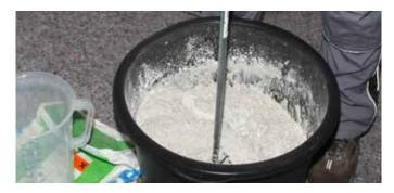
2 KÖSTER Hydrosilicate Adhesive SK is mixed with approximately 5.2 liters of water using a slowly rotating electrical mixer into a homogenous consistency.
