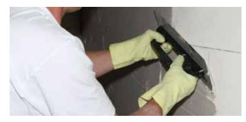
Afterwards, the whole area is plastered with a layer of KÖSTER Hydrosilicate Adhesive SK in a maximum thickness of 2 mm.
