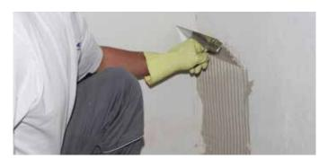
The adhesive is then applied to the substrate with a 8 mm notched trowel, fully covering the board area.
