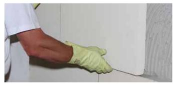
A Next, the KÖSTER Hydrosilicate Boards are pressed onto the wall and leveled. The boards and the butted joints must be completely glued.
